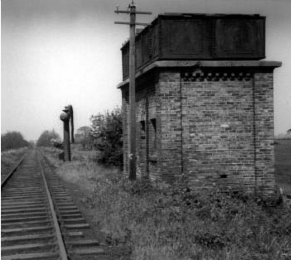
At the Chevington end of Amble's branch line stood a water tower and crane.
